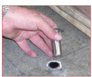
well as around it. Using mallet, tap rubber insert into hole. Next place the carrier support receptacle in the hole and strike with rubber mallet until metal flange is flush with the floor.
